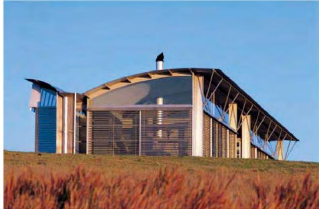
**Glen Murcutt's South Wales house collects and funnels water through the roof's central groove.**
