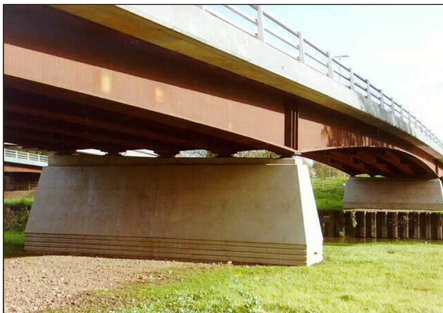
Sumber: courtesy of Corus - Westgate bridge, Gloucester
