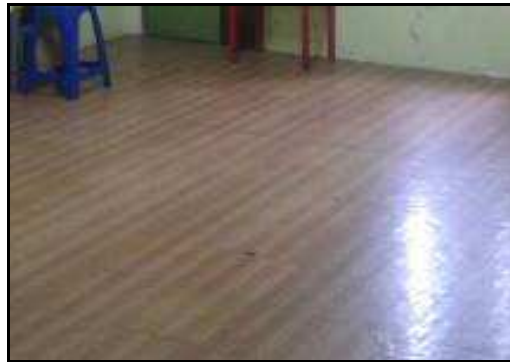
Gambar 2.37 Lantai Kelas Nursery One – Two – Three
