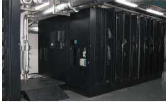
*Gambar 2.12 Row-cooled CACS (Schneider Electric, 2013)*
