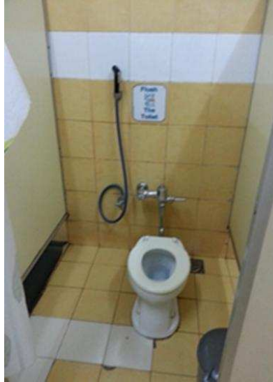
Gambar 2.133 Toilet Santa Laurensia 2
